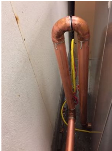
Drainage - 2 feet upwards, then downwards
